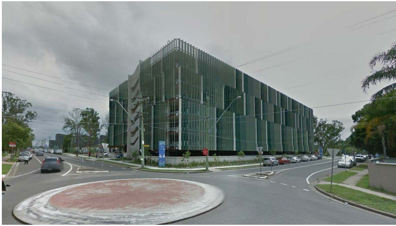
CNR. SOMERSET ST / DERBY ST NEPEAN CAR PARKING COMPLEX 8 STOREYS
