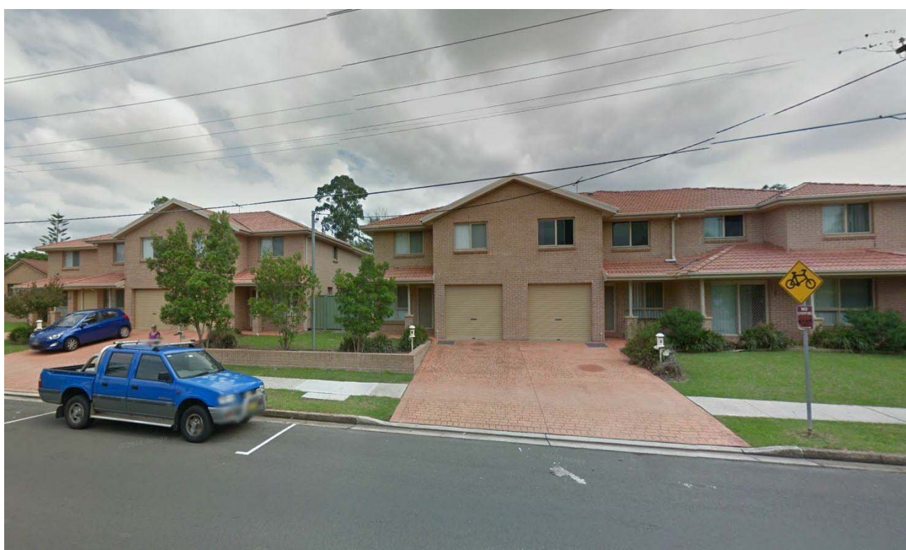
29-33 SOMERSET ST 2 STOREY RESIDENCES BRICK CLADDING, TILE ROOFING
